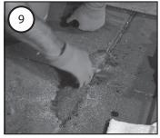
With a wide putty knife or trowel, scrape or trowel the surface smooth and/or level it with the surrounding concrete. (A final sprinkling of sand may be needed for added traction.)
