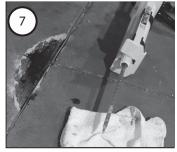
It is important to always keep your cartridge pointing downward or horizontally to prevent the Flash Floor mixture from flowing back into the cartridge.
