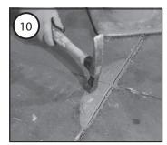
Allow 15 - 30 mins (depending on the ambient temperature) for Flash Floor to harden. Repairs made in Cold Storage can take much longer to harden
