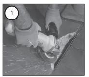
Clean the surface of the repair area with an angle grinder or chipping hammer. Other tools may be used as long as they clean the surface and expose the pores of the concrete.
