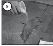
Lightly sprinkle sand over the repair to soak up excess Flash Floor.
