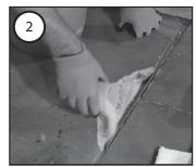
Fill your repair area with 100% dry sand. If your area is deeper than 1 - 2 inches then fill it 1 - 2 inches at a time and repeat steps 6 and 2 until the repair area is filled.
