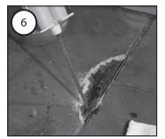
Saturate the sand with Flash Floor, let it settle for 3-5 seconds, and repeat until it pools at the surface. Cracks or voids may cause drainage. Watch the "Creating A Seal" video for preventing
