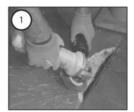
Clean the surface of the repair area with a wirewheel attachment and grinder. Other tools may be used as long as they exspose clean concrete.
